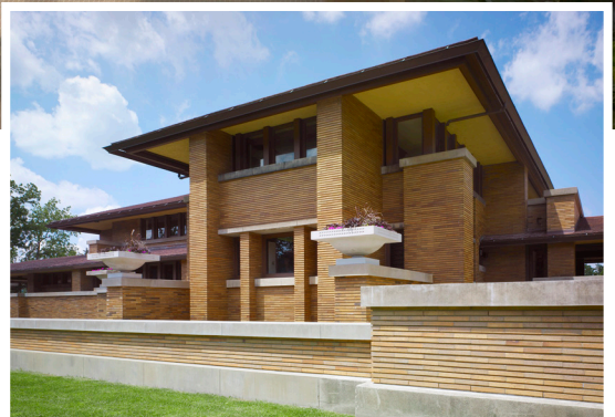
Above: The conservatory at the Darwin D. Martin Complex House; the main house features Wright's characteristic cantilevered roof.
